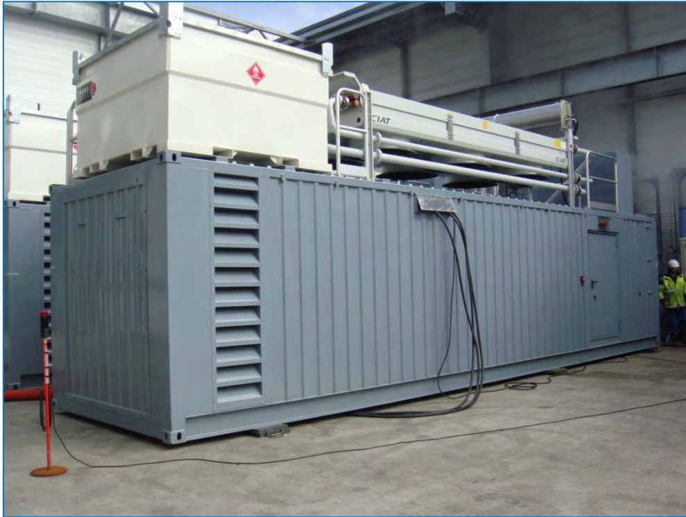
Figure 2-1: Emergency diesel generator (QSK78)
