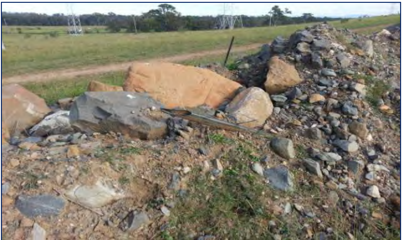
Photograph 2. Fill materials along the western boundary of the site.
